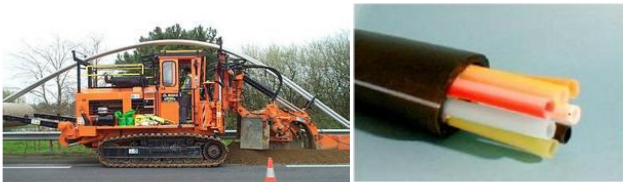
Figure 7: Trenching machine and duct containing multiple subducts
