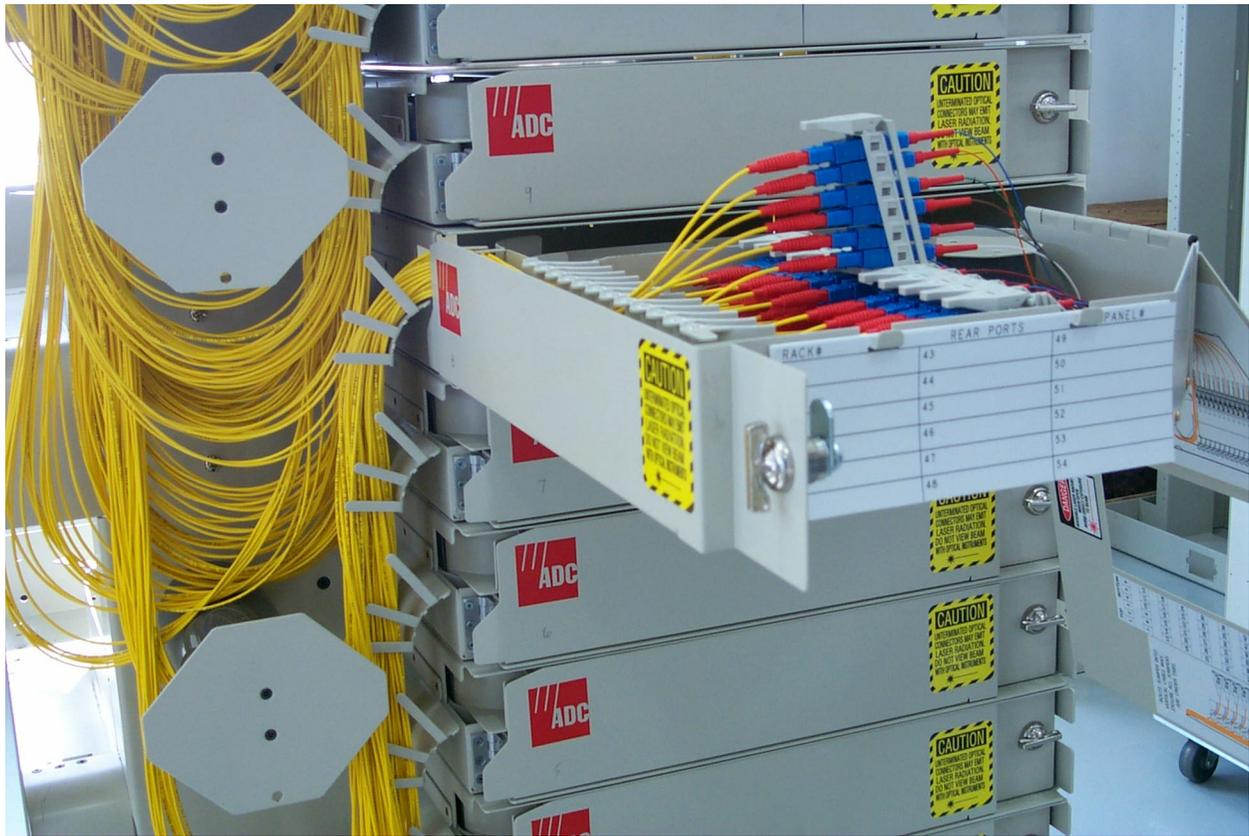
**Figure 10. Installed Connectors**
