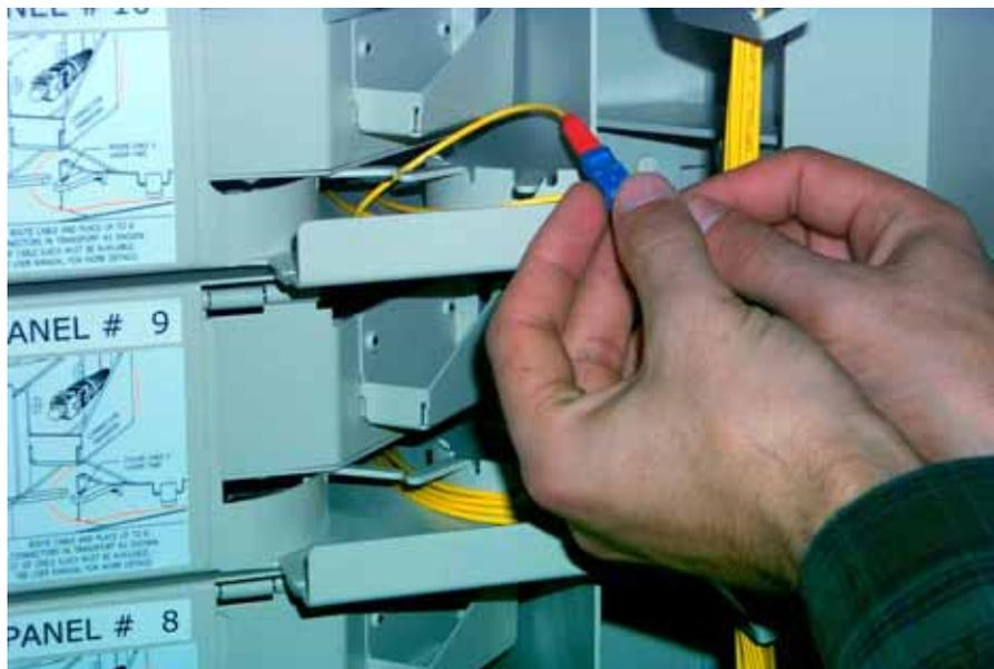
**Figure 55. Positioning Patch Cord in Radius limiters**
