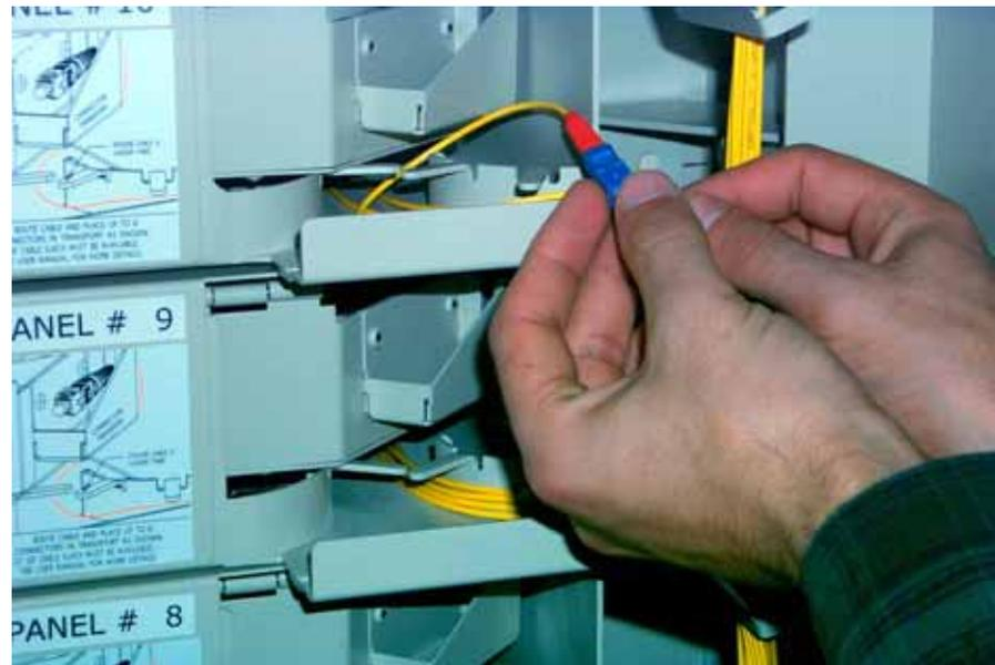
**Figure 45. Positioning Patch Cord in Radius Limiters**
