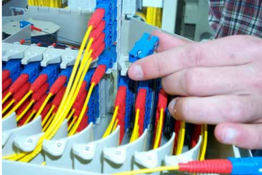
**Figure 77. Removed Adapter**
