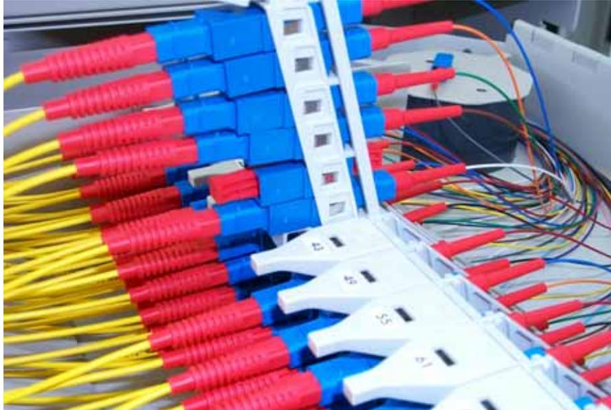
**Figure 79. Installed New Adapter**
